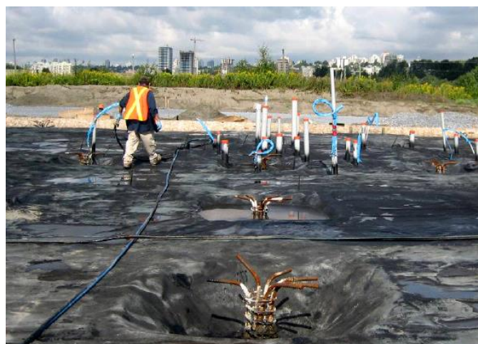
Photograph 02 – Installation of asphalt barrier
